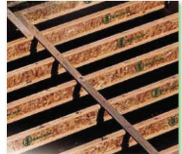
BCI® Joist top flanges must remain straight within a tolerance of 12mm from true horizontal alignment and within a tolerance of 3mm from true vertical alignment.
